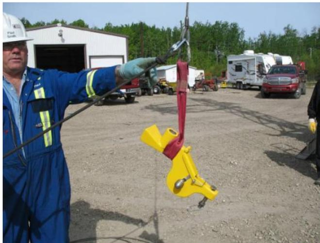
2.3.1.3. Fasten a hoisting sling securely around the docking station, attach the assembly to the winch & tag line. (If mounting the docking station without the cable proceed to 4.2.3.)
