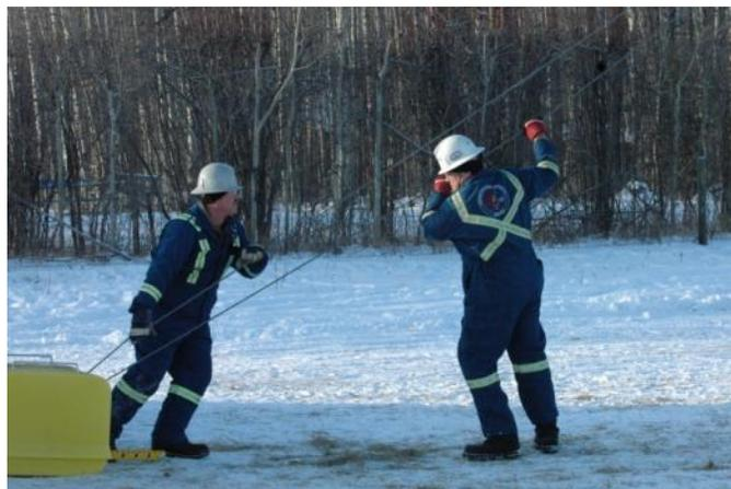
2.11.2.1. Pulling the lower cable towards the Magnegress & pulling the upper cable towards the docking station will propel the trolley up to the person at the docking station waiting to guide it into place.
