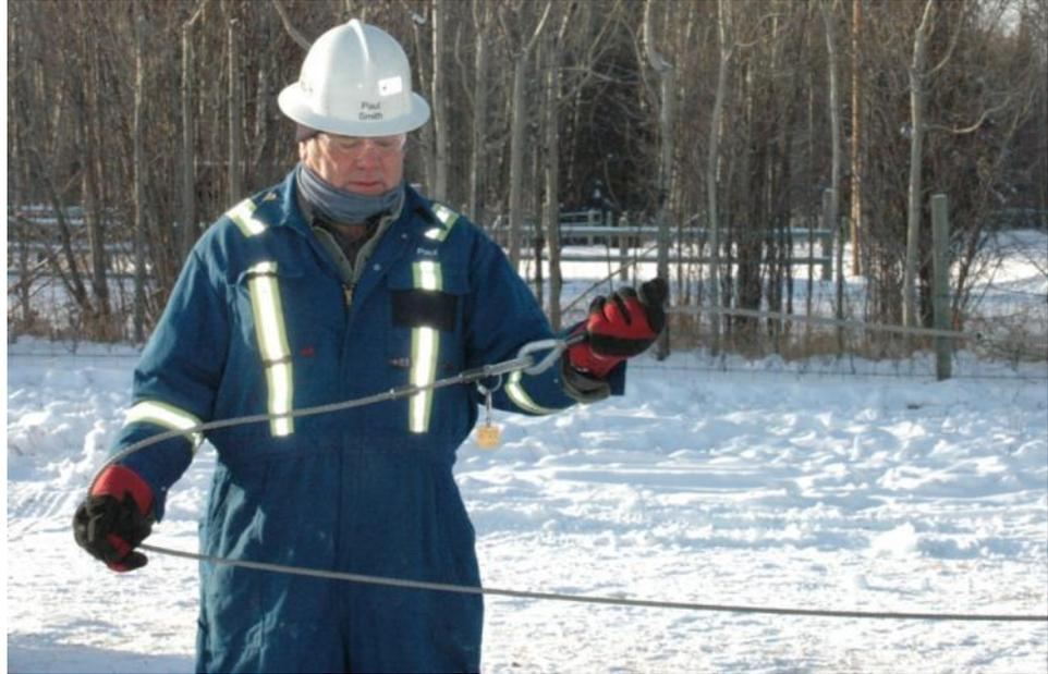
2.7.3. Keeping the cable separated grasp cable firmly & walk towards the desired anchor position.
