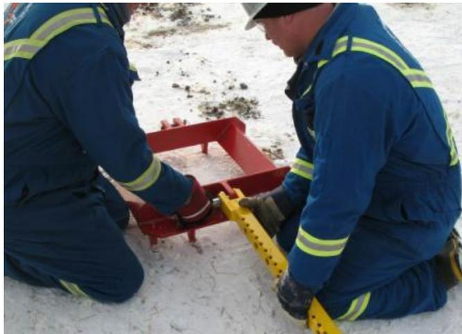
2.5.1. Position the Bear Claw park-on anchor so it attaches to the tension link & install anchor bolt through tension link. Install nut & safety pin.
