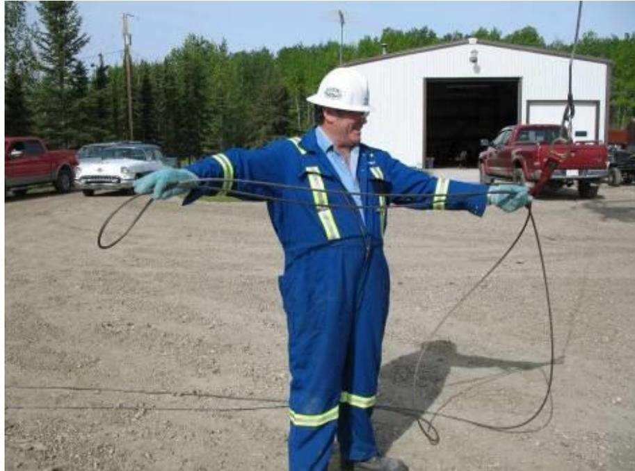
2.3.2.3. Fasten a hoisting sling securely to the cable leaving approximately 6 ft (2.8 m) of tail.
