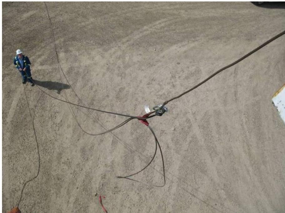
2.3.2.4. Winch the cable to the docking station.
