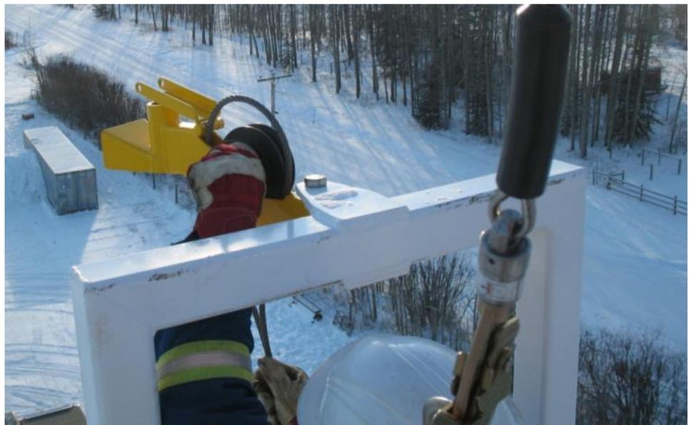
2.3.2.12. Insert sheave inside the 180° back bend & line up the flats on the sheave shaft to the slots in the docking system.
