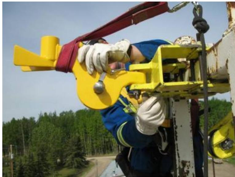
2.3.2.1. Mount the docking station to the platform's mounting point. Use the supplied bolt & safety pin.
